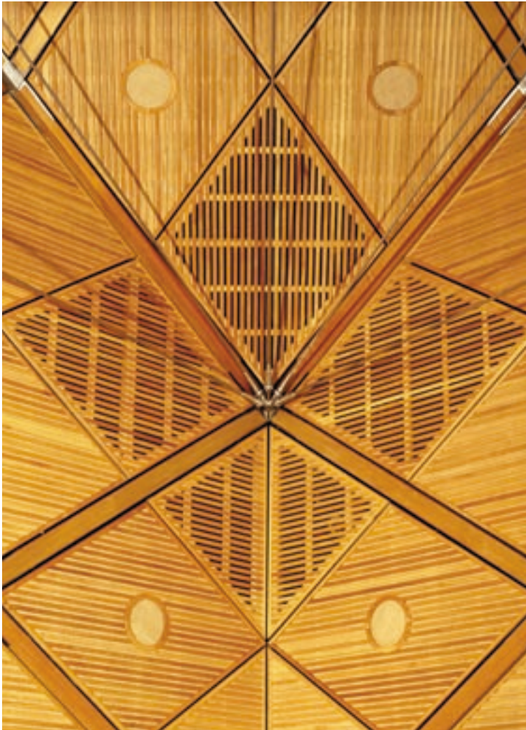
Haberdasher's Hall, London, uses American white oak to blend traditional materials and building techniques in a 21st century venue. Architect: Michael Hopkins and Partners. Client: Haberdasher's Company.
